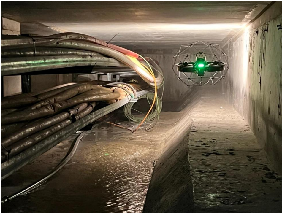
© Flyability – Mapping de 13 km de galeries techniques
