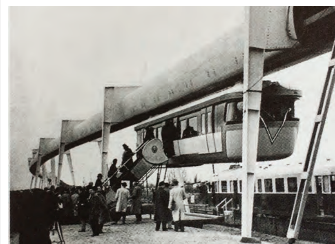
Fig. 4 – Essais du monorail en 1960 (Source: Gil et Pleutin ©Editions Sutton 2013) Fig.4 – Testen van de monorail in 1960 (bron: Gil et Pleutin ©Editions Sutton 2013) Fig.4 – Monorail trials in 1960 (Source: Gil et Pleutin ©Editions Sutton 2013)
